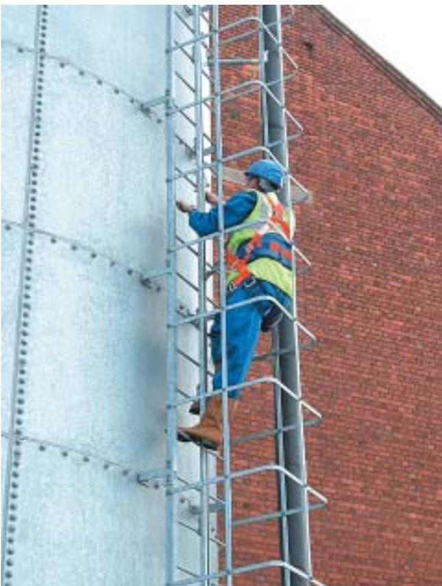
A12 Safety Rail installed to existing ladder.
