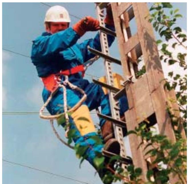
A12 Double Rung Ladder used for maintenance on a floodlight tower
