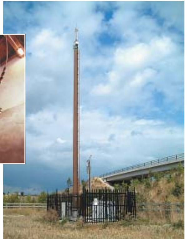
Invisirung™ fitted to a Dynamic Concepts timber monopole
